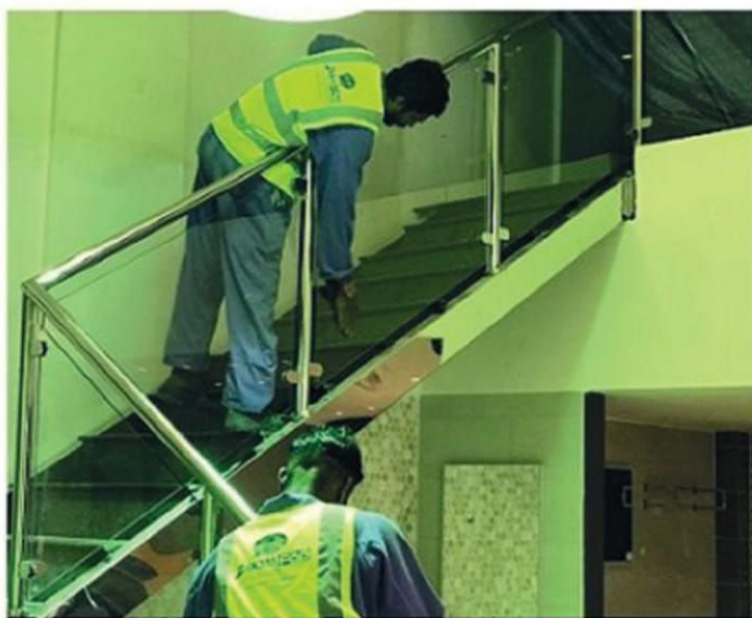
30. Project : Renovation of Office @ Salwa Road Scope : Steel Stair with SS Handrails and glass Balustrades
