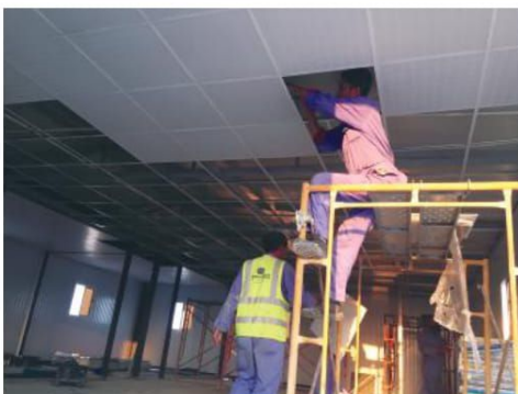
27. Project : Smeet Ready Mix Lusail Office. Scope : Office room Gypsum ceiling Works
