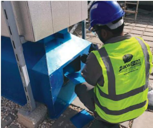
24. Project : NPP- 0076 Ocean Blue –New Port. Scope : Aluminum Flashing Cover around Parapet and Duct
