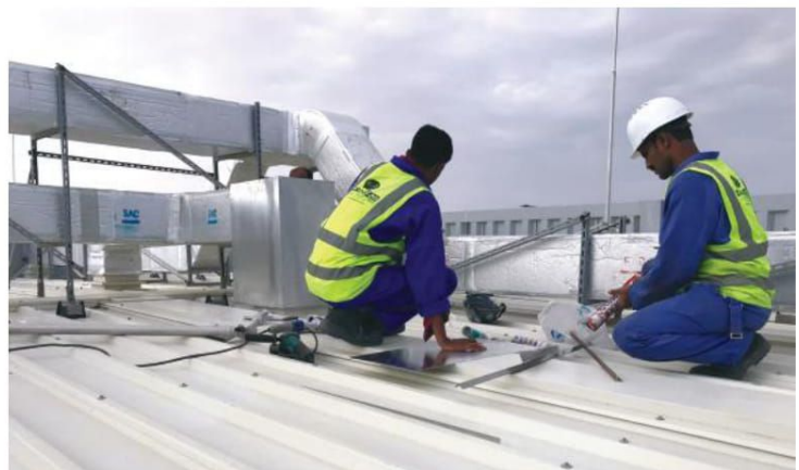
21. Project : NPP- 0076 Ocean Blue –New Port. Scope : Aluminum Cover around Ducting
