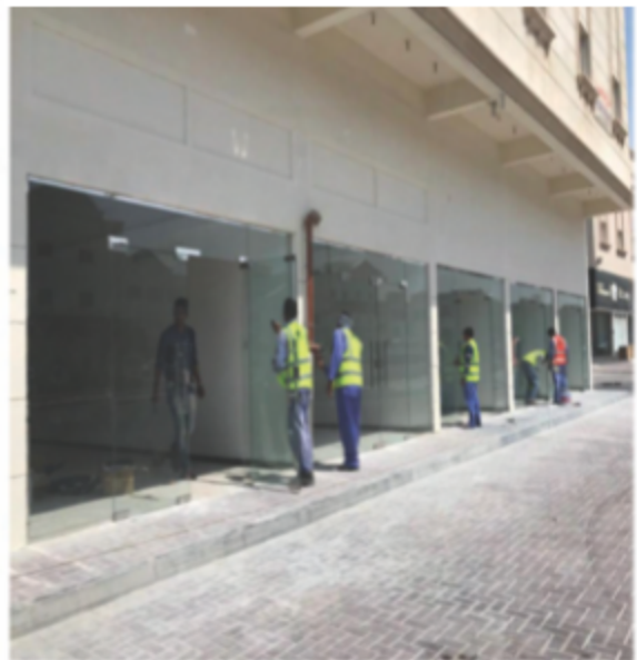
Project : Rayyan Zaatar. Scope : Shop front glass Partition and Door
