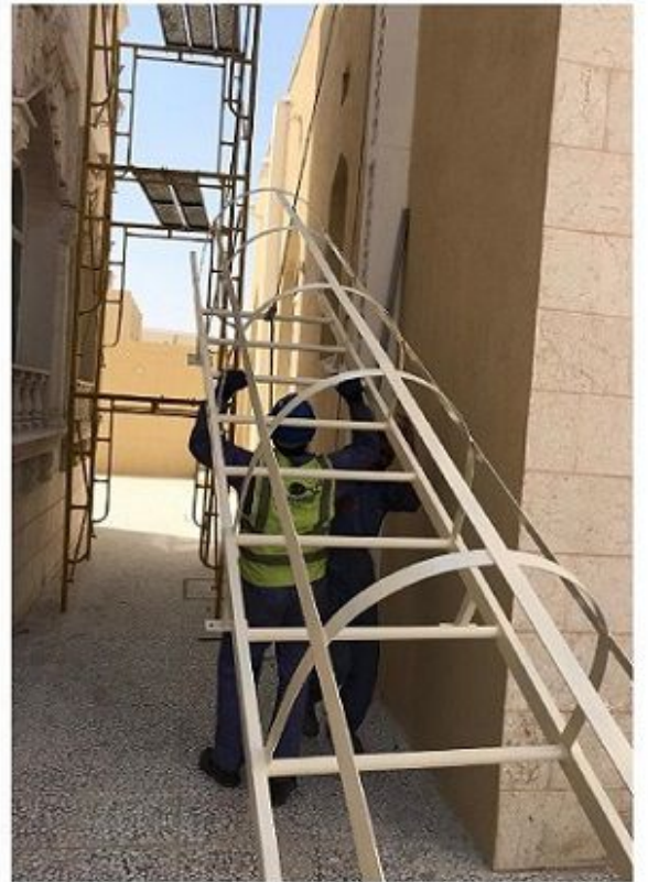
38. Project : 6 + 2 Construction of Villa @ Sailiya Scope : Caged Ladder for Majlis
